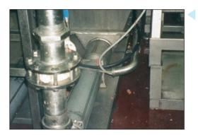
A customer, producing mechanically deboned meats, which are frozen before export to food manufacturers worldwide, has installed a stainless steel W062 pump. The meat puree is gravity fed into the inlet hopper for transfer to the freezer plates. The efficiency of the freezing system relies on a constant flow rate of 5 tonnes per hour, to prevent the plates standing idle or a delay further up the line.
