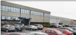
Montreal, Canada Velan Inc., Plant 5
