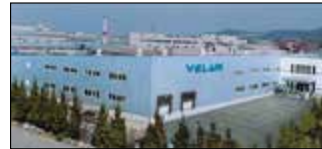
Ansan City, South Korea Velan Ltd., Plant 2
