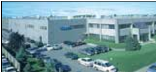
Montreal, Canada Velan Inc., Plant 2 and 7
