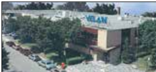
Montreal, Canada Velan Inc., Plant 1
