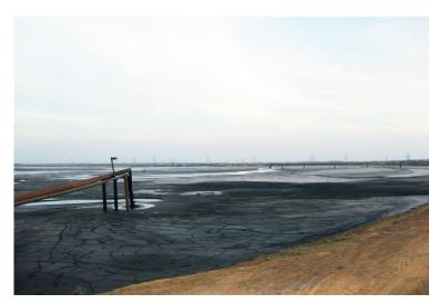
Ash dyke - an ABEL HMQ pump conveys the ash slurry with 65% concentration to this spot 7.5 km away - with such little water content the dry ash solidifies in 3 to 5 hours
