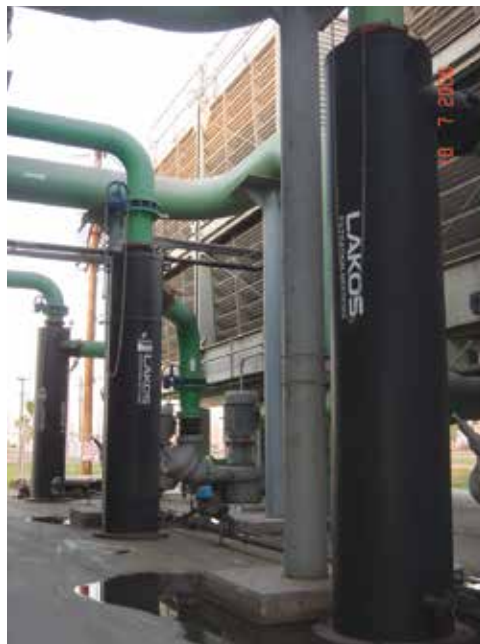
Series of LAKOS HTH 1950 separators used to keep sand out of customer cooling tower installation in Mexico.
