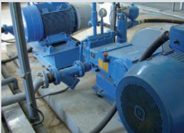
Electro-pneumatically actuated ABEL 3/2-way bypass valve
