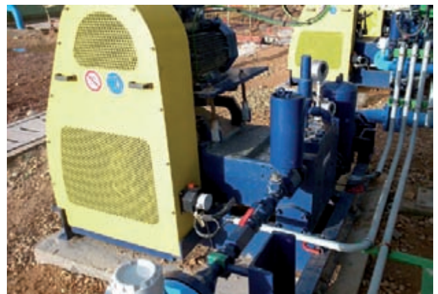
ABEL HPT-K-32 to supply gland water to up to 5 centrifugal pumps in parallel
