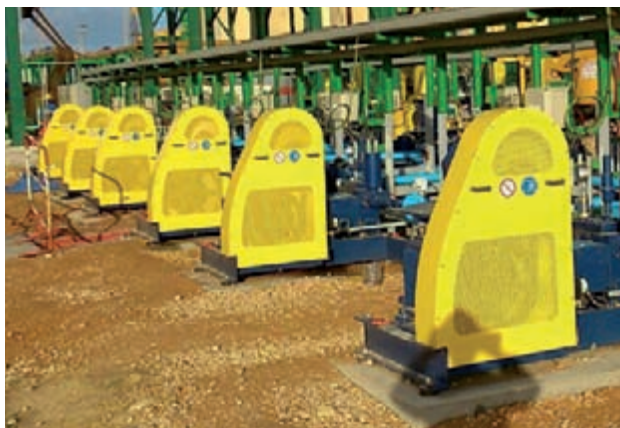
ABEL HPT gland seal water pumps on a phosphate mine in North Africa
