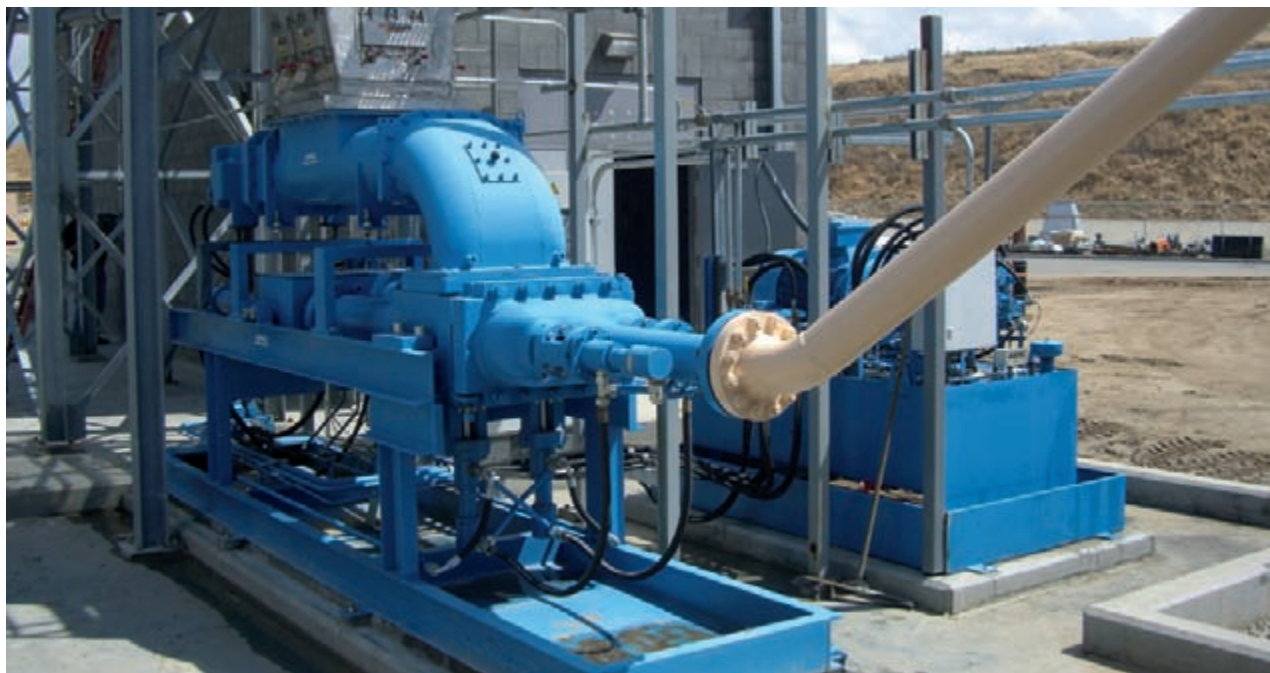
ABEL Solids Handling Pump unit with hydraulic power pack and twin screw feeder
