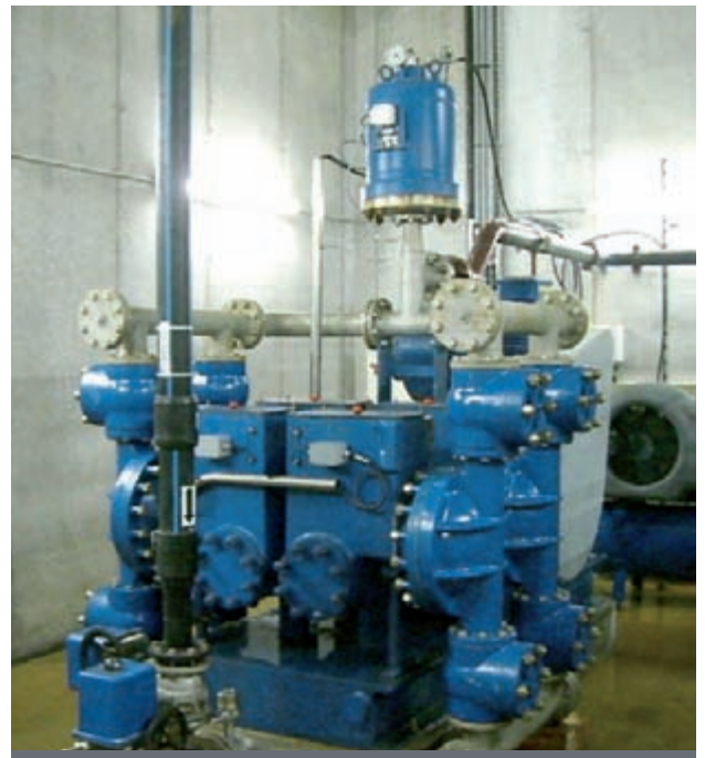
ABEL HMQ in a saline application for backfilling of brine slurry with 30 % solids concentration
