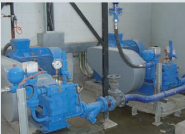
ABEL HP-K-25 for filter cloth cleaning of chamber filter presses
