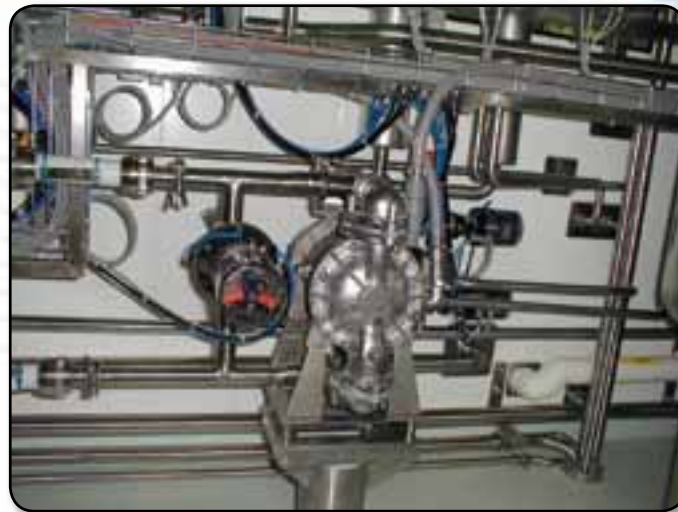
USDA certified ball check valve pump in a clean-in-place, sanitary piping installation.
