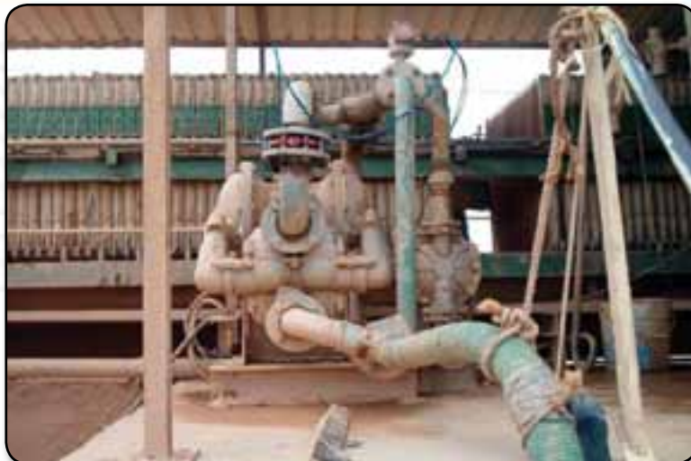
3" HDB bottom ported pump installed as a plate & frame filter press, pre-coat supply pump.
