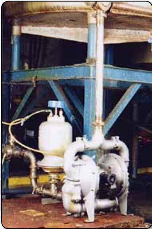
Heavy duty flap valve pump installed on an underflow sludge transfer application.
