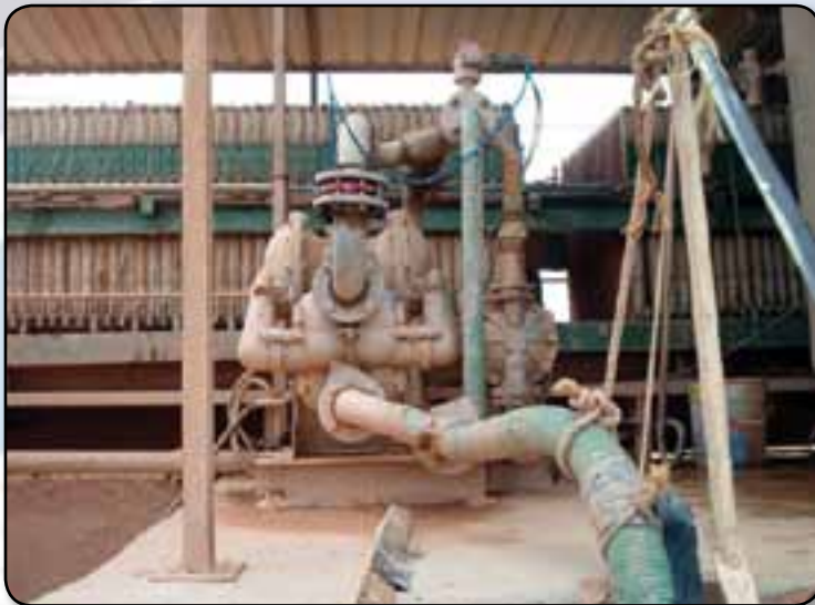
Custom built heavy duty wastewater, filter press pumping system.
