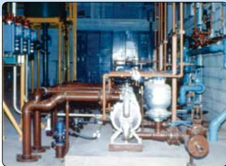
Heavy duty flap valve pumps with tranquilizers permanently installed in an automotive industrial waste treatment facility.
