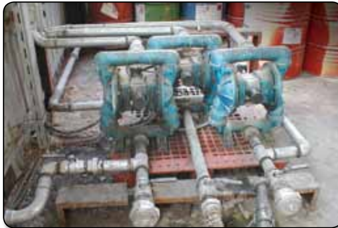
Metallic standard duty pumps installed for exterior sump pumping requirements.
