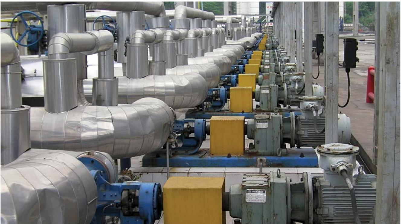
*Viking Internal Gear Process Pumps at a Chemical Plant.*
