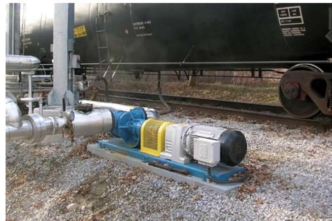
Viking internal gear pump in a railcar unloading application.
